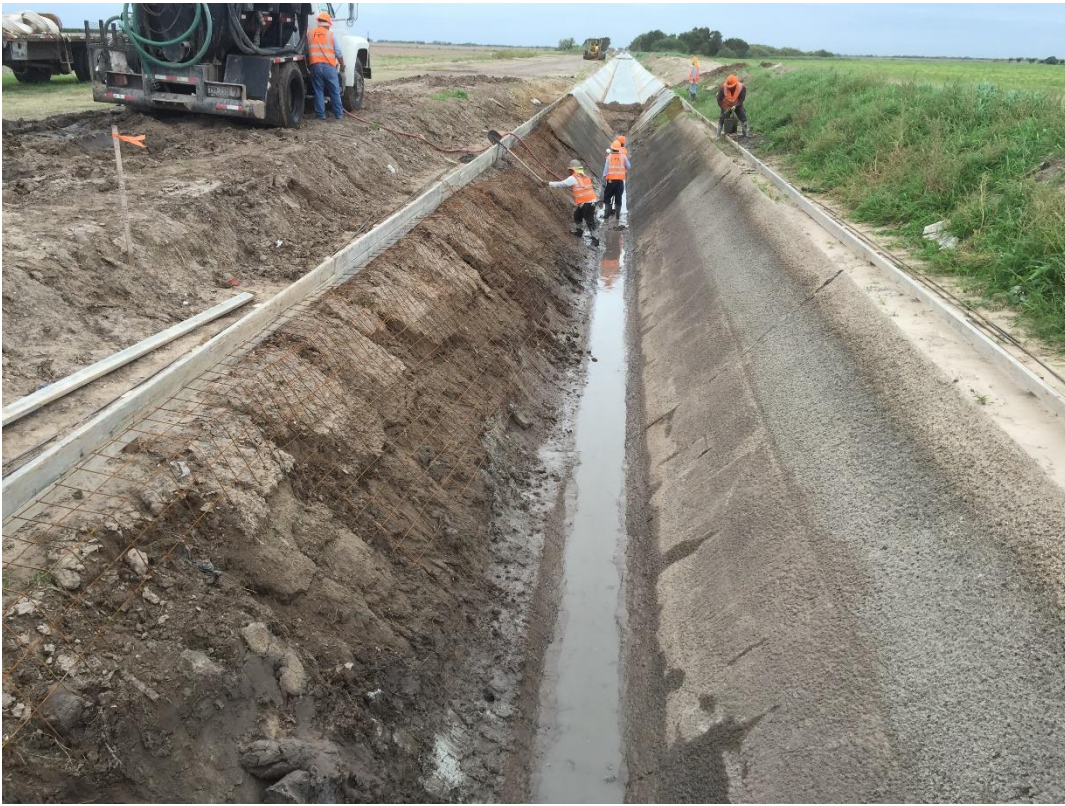
Figure 13 Preparation of Phase I Canal for shotcrete.
