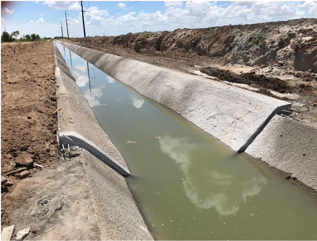
Figure 21 Completed Phase II Canal.
