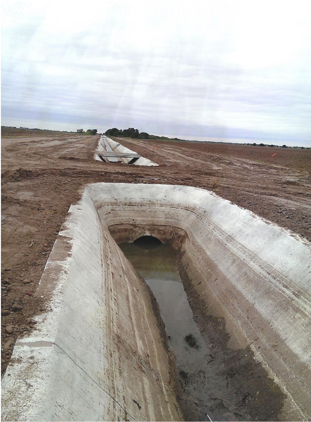
Figure 18 Completed Phase I Canal.
