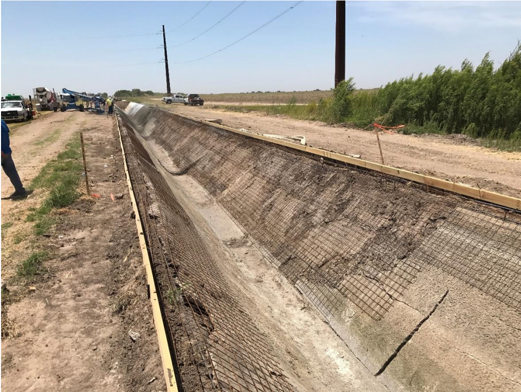
Figure 19 Phase II Canal prepared for lining.
