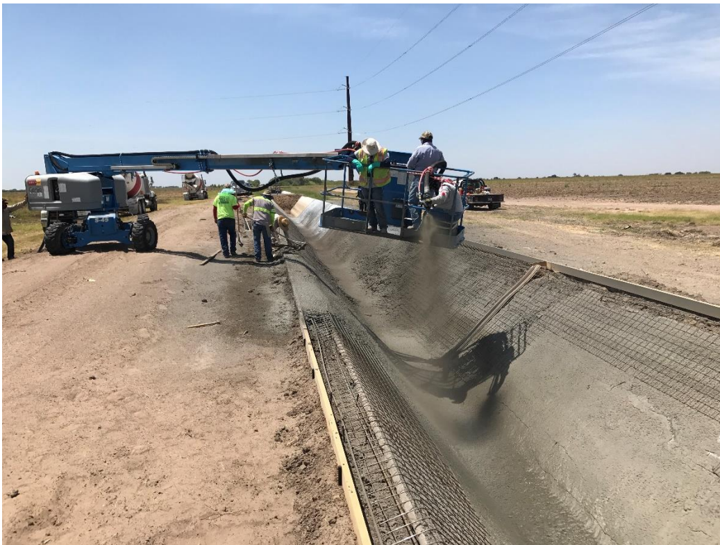
Figure 20 Southern Trenchless applying shotcrete.
