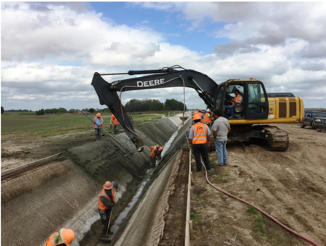
Figure 14 Phase I shotcrete application.
