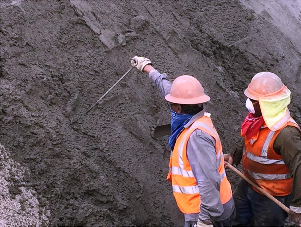
Figure 15 Shotcrete thickness gauge.
